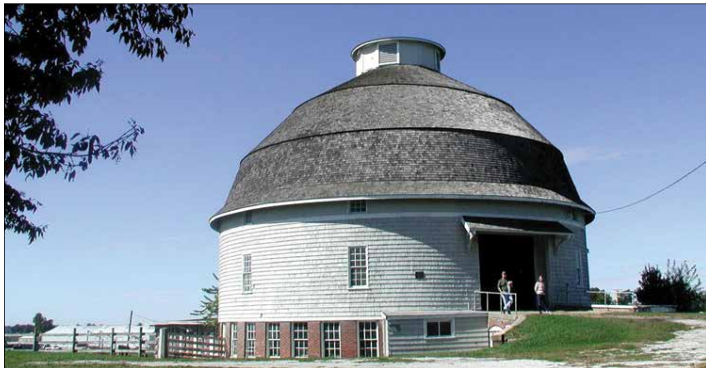
Figure I.10: One of the three University of Illinois round experimental barns, 70 feet in diameter (shown on the left side of the aerial photo in Figure I.9). The dairy cows are cared for on the lower level and the hay and silage are brought in on the upper level.
