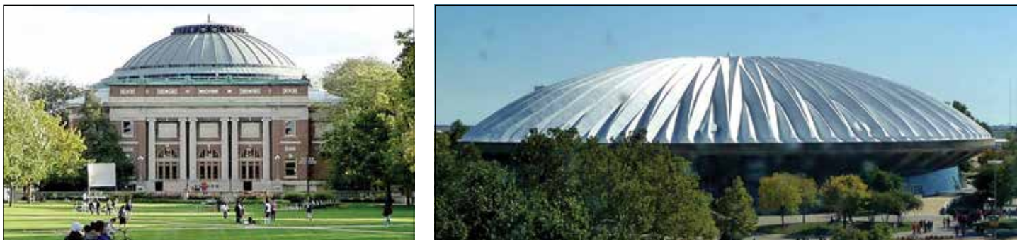
Figures I.20 and I.21: On the left, the University of Illinois' Foellinger Auditorium rotunda, and the "flying saucer" arena (now named the State Farm Center), in Champaign, Illinois.
