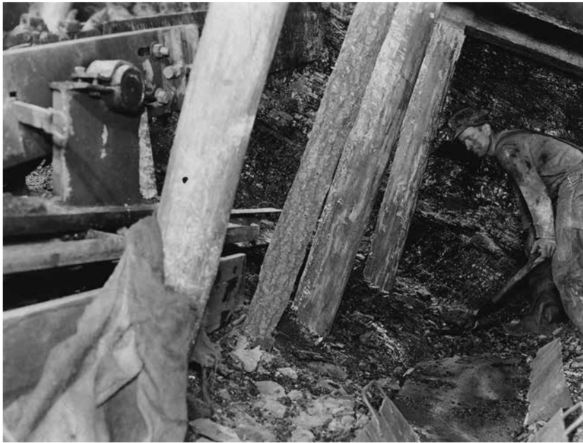
Cle Elum miner Art Pasa shovels coal onto a jig conveyor in No. 5 mine in 1942. A vertical coal cutting machine at rear left was designed and built by Northwestern Improvement Company engineers and mechanics in Roslyn to accommodate the steep sloped conditions in the mines. Courtesy of Roslyn Public Library, Roslyn Heritage Collection, by permission of Frank Schuchman
