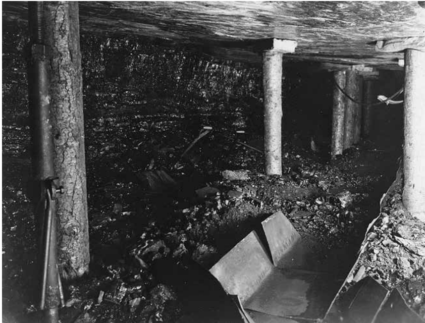
A typical workplace for a coal miner inside Roslyn's No. 5 mine. Miners in 1932 were completing a cross cut between entries in this mine when a coal-cutting machine hit a pocket of gas and sparked a fire. Five miners eventually died from their burns. Courtesy of Roslyn Public Library, Roslyn Heritage Collection, by permission of Frank Schuchman
